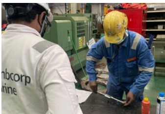
Performing portable machine drilling and tapping
