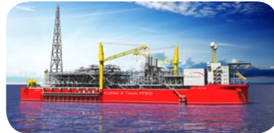
Energean Power FPSO for Karish Field Development
